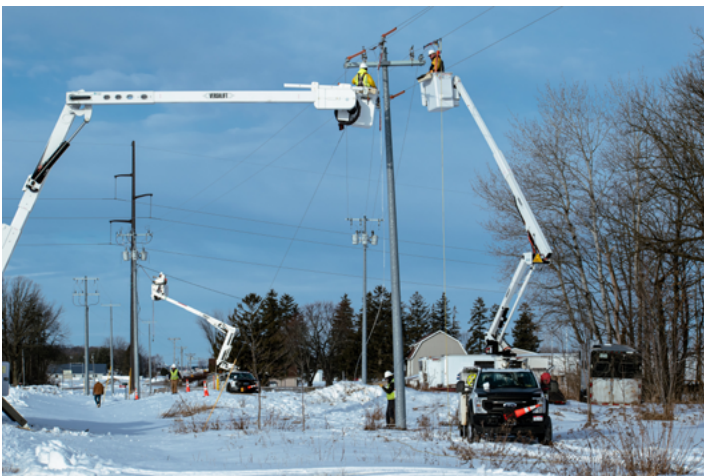
Overhead electric line replacement
